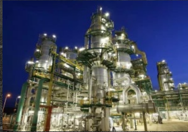
Repsol Petroleum Plant – Constanti Spain
